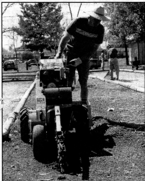
Jacques Mathieu starts to cut a trench for the irrigation lines.
